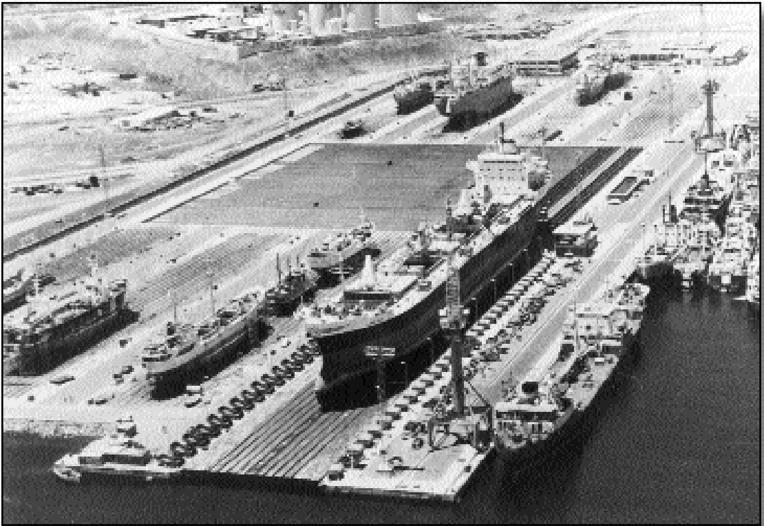
Astilleros Canarios, S.A., Las Palmas, Canary Islands Syncrolift® dimensions: 171.6m long x 30m wide; capacity: 28,000 DWT
